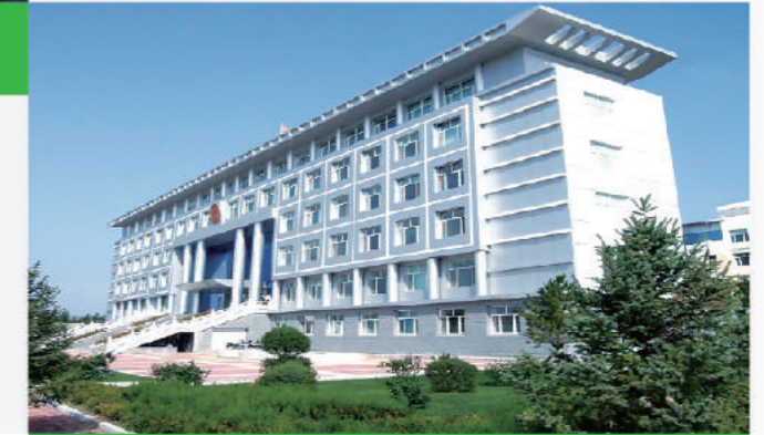
Government building in Inner Mongolia , China.
