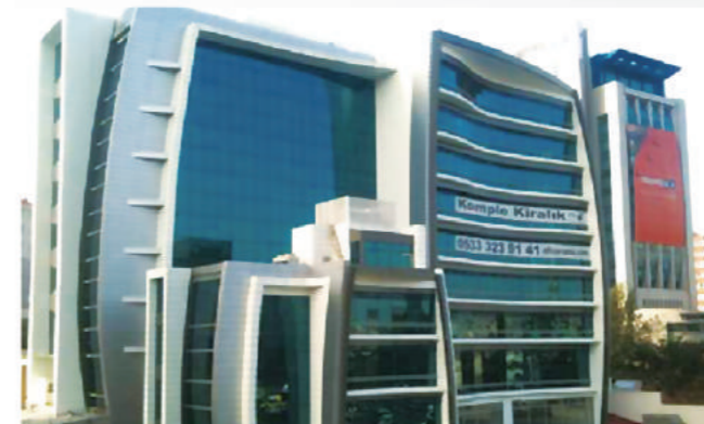
Office building in Istanbul, Turkey.
