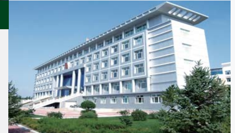
Government building in Inner Mongolia , China.
